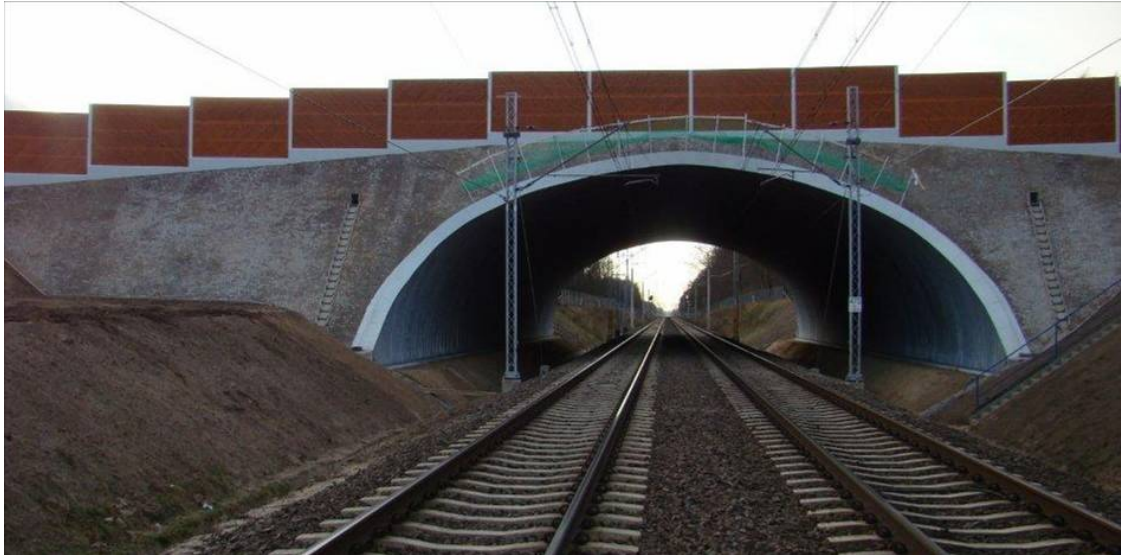
Figure 2.2 By completing the steel structure with well-designed details, nice looking bridges can be achieved. This bridge is one of the largest SSCB in Europe having a 20 m span.
