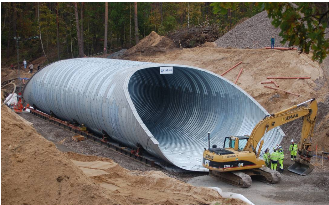
Figure 2.1 The finalized erection of the steel part of a SuperCor horizontal ellipse bridge, see Figure 1.3 B, just before starting the backfilling process.
