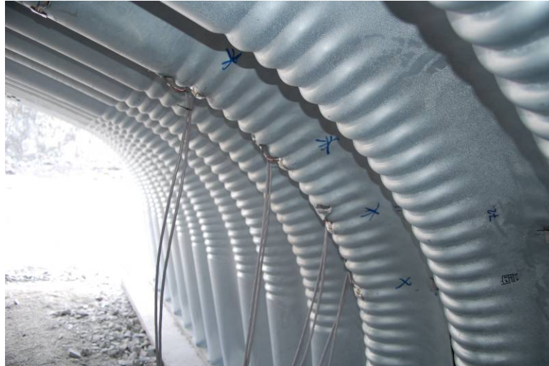
Figure B1.1 Photo showing so called cross corrugation (from the Järpås full scale tests).
