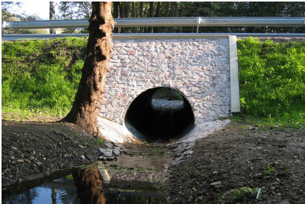
Figure 2.3 A nicely worked out glacis covering the slopes of a pipe-arch bridge.
